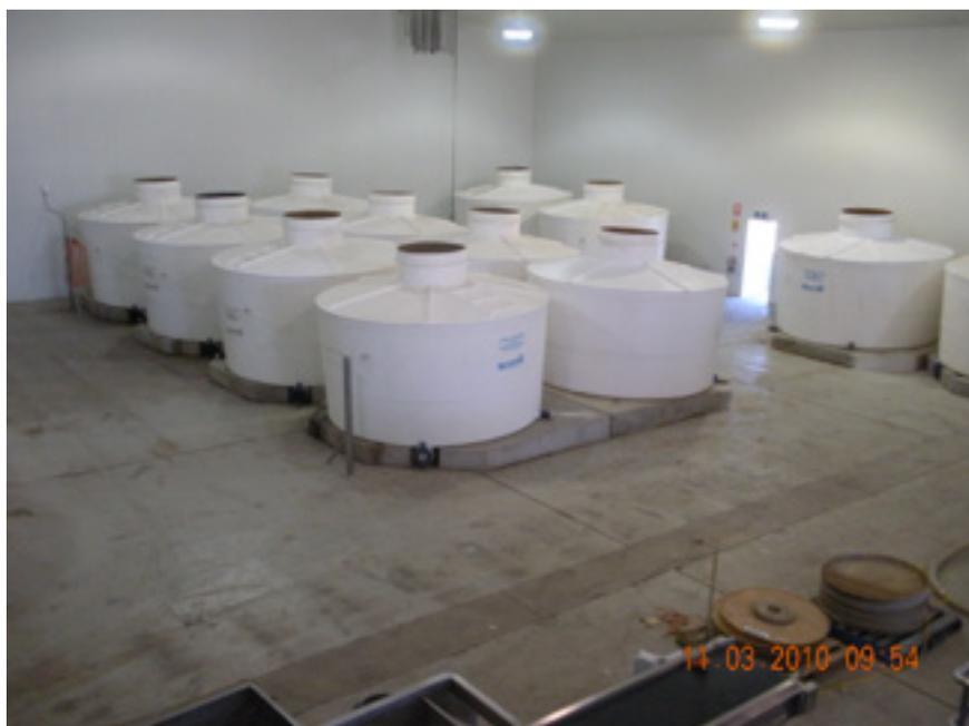
**Figure 1:** New FRP tanks on sloping plinths being fitted out. Note power line on left-hand-side of tank.
